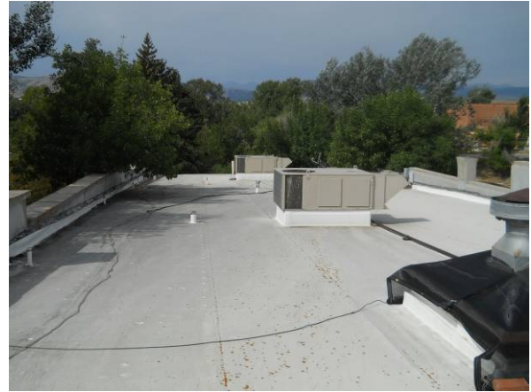
South building roof looking west
