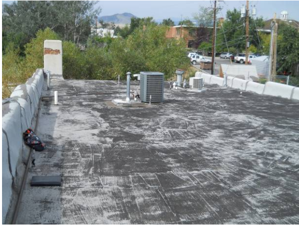
North building roof looking west
