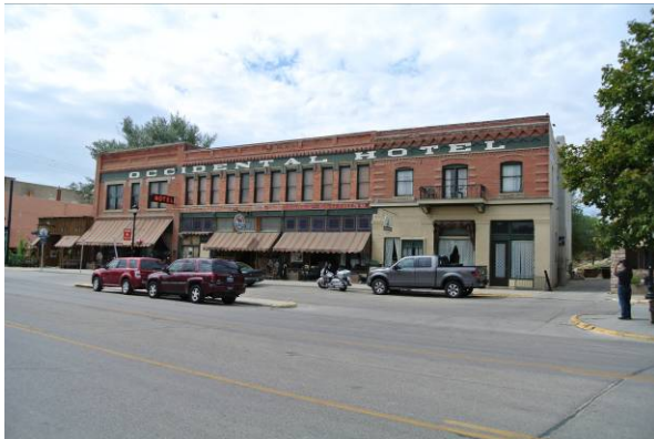
East façade from northeast
