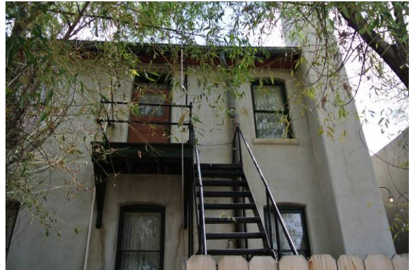
North building, west façade
