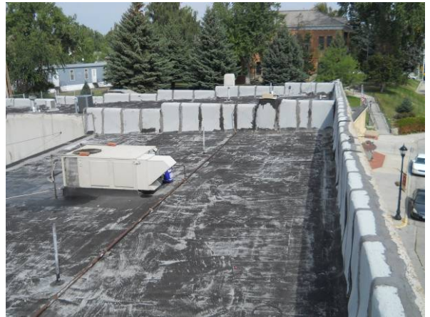
Upper middle building roof looking north
