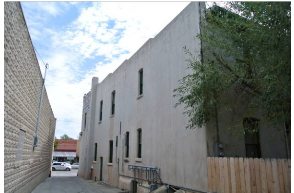
North façade from northwest
