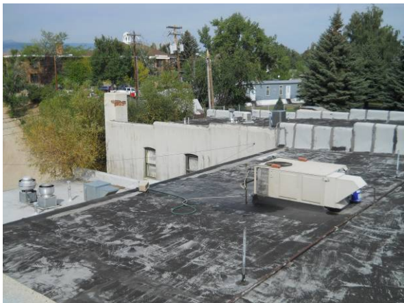
Upper middle building roof looking northwest
