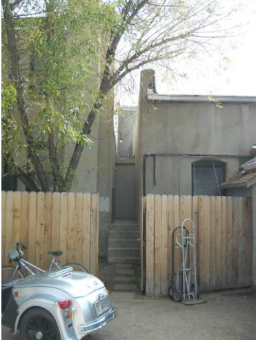
North building west access stair
