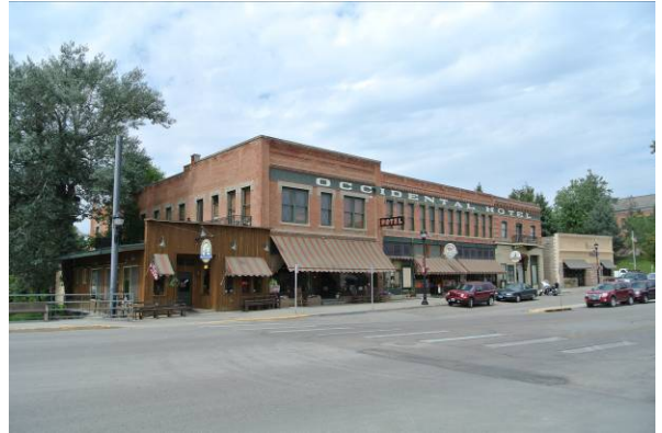
East façade from South Main Street and Fetterman Street
