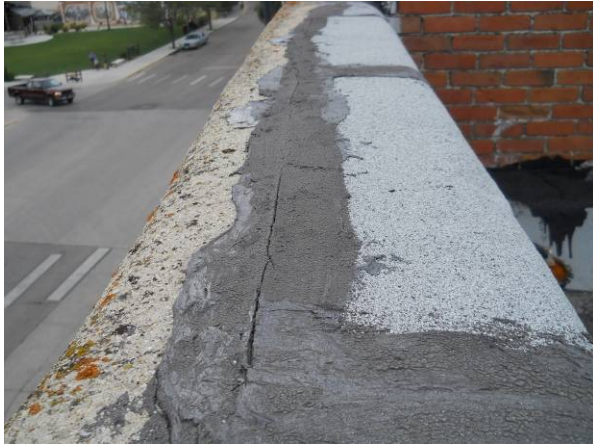
Roofing membrane termination at parapet coping on middle building roof
