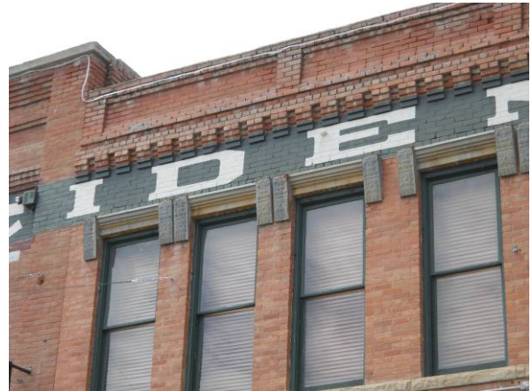
Middle building east parapet/cornice detail
