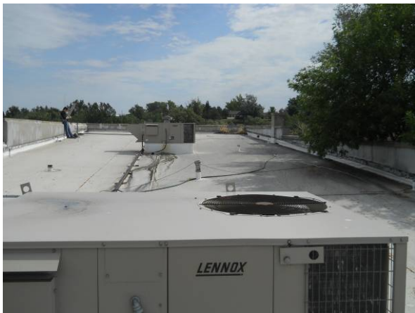
South building roof looking east
