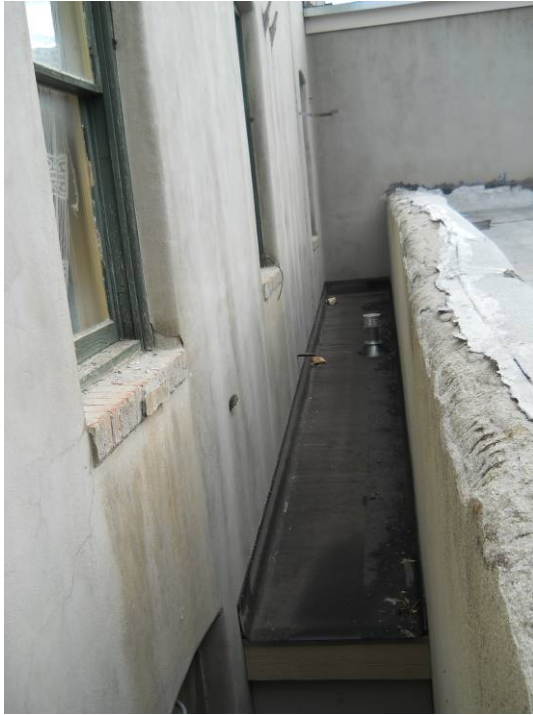
Trough gutter between north building roof and lower middle building roof
