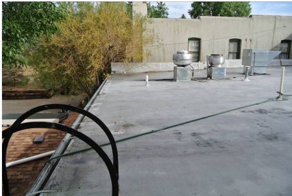
Lower middle building roof looking north
