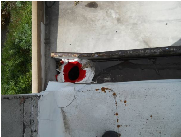
South building roof gutter/downspout connection
