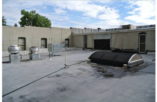
Lower middle building roof looking northeast
