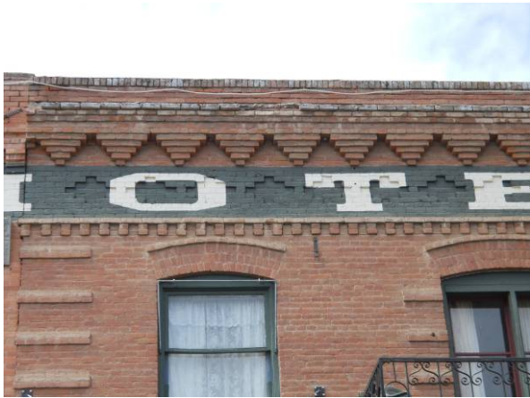
North building east parapet/cornice detail
