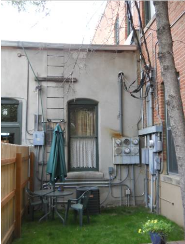
Roof access on west facade, middle building
