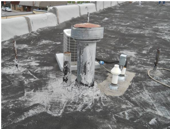
Typical rolled roofing membrane roof penetrations
