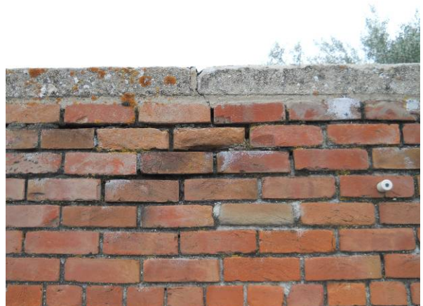
Typical mortar joints on south building roof
