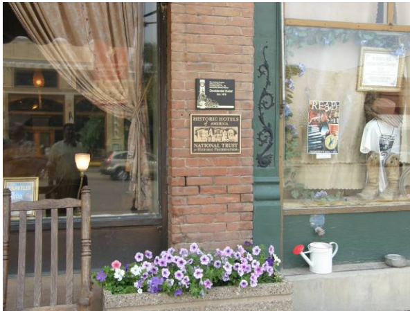
North building, east facade, historic designation hotel plaques
