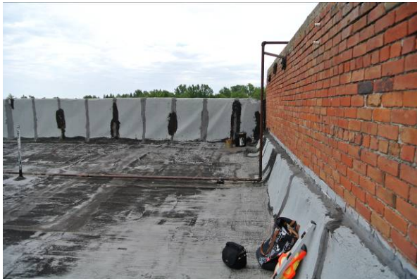
Gas line from south building roof to upper middle building roof
