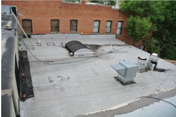
Lower middle building roof looking southwest
