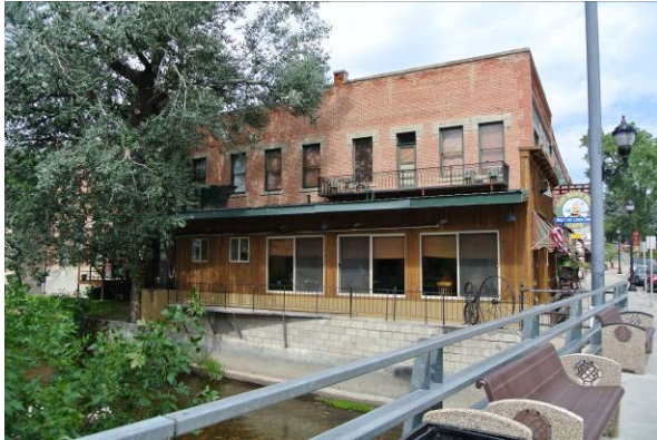
South façade from corner of South Main Street and Fetterman Street
