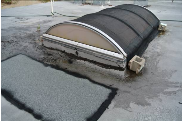
Skylight on lower middle building roof
