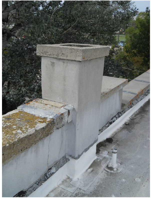
Typical parapet/cap/chimney construction on south building roof
