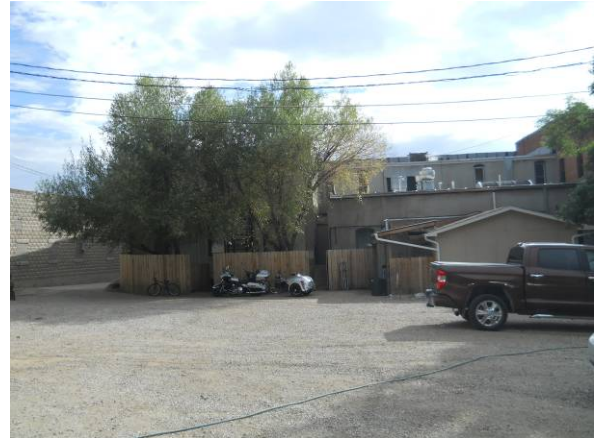
View looking east (back of building), north and middle buildings
