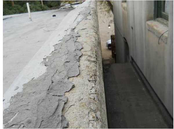
Lower middle building roof curb/parapet on north side
