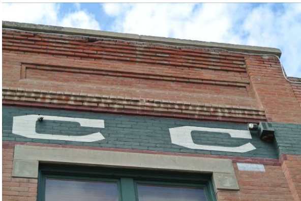
South building east parapet/cornice detail
