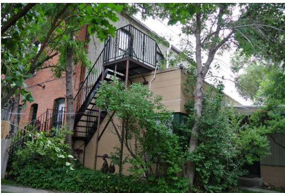
South building with addition, view from northwest
