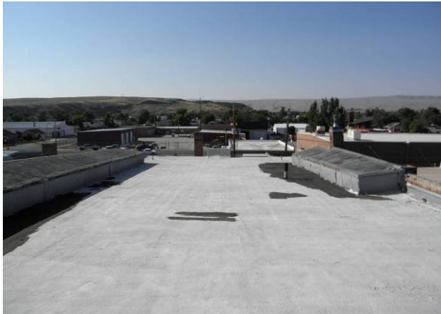
Upper roof looking south
