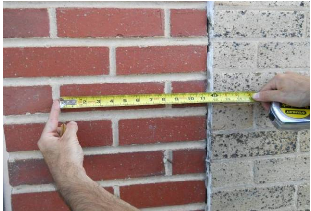
North façade brick
