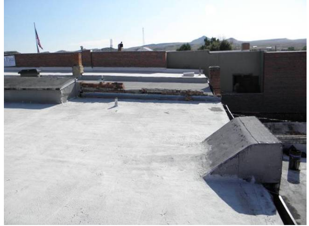
Upper roof, looking east
