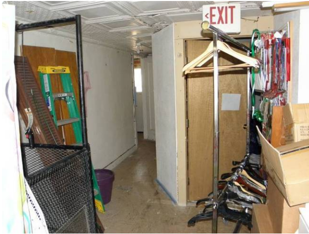
Back of under mezzanine looking south, storage & south stair to basement beyond
