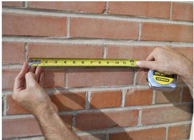
South façade brick
