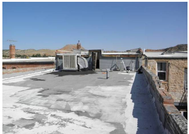
Lower roof looking northwest
