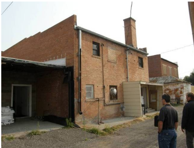
Southwest corner looking Northeast
