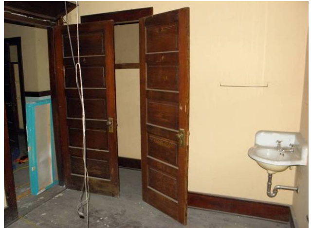
Room #4 looking northwest, entry corridor beyond
