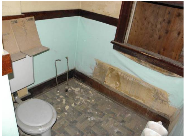
Bathroom interior view looking southwest
