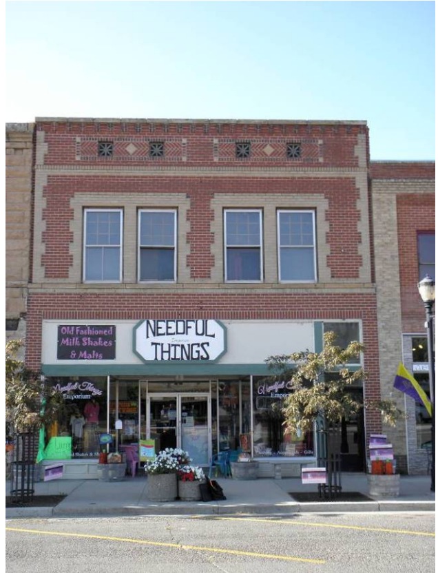
North façade looking South
