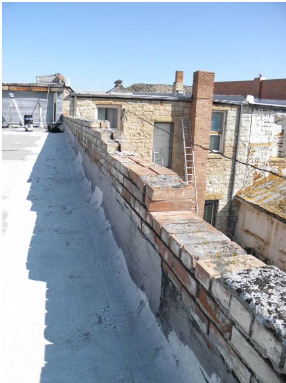
View of lower east brick parapet
