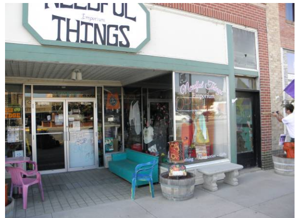
View of storefront, west door to second floor and transoms above
