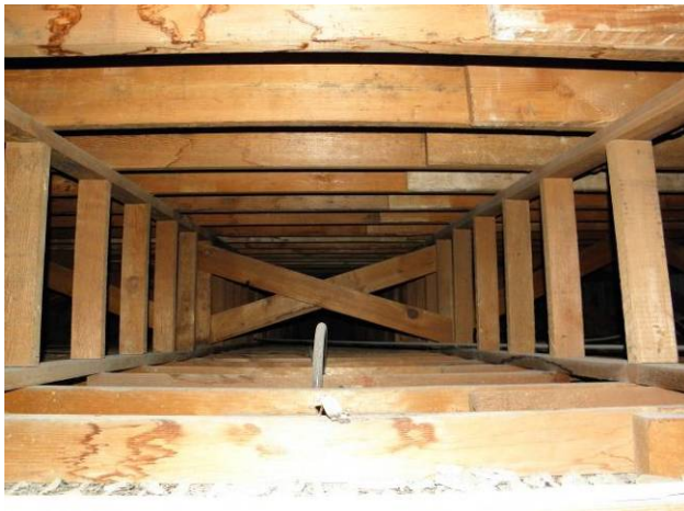
Attic space above corridor at south end – looking north
