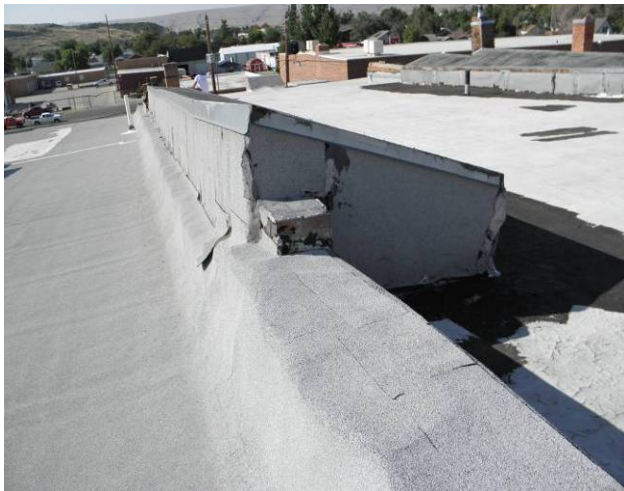
View of east lightwell looking southwest
