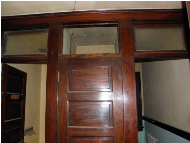
Transom windows above entries to single restroom, utility sink, and bathroom (left to right)
