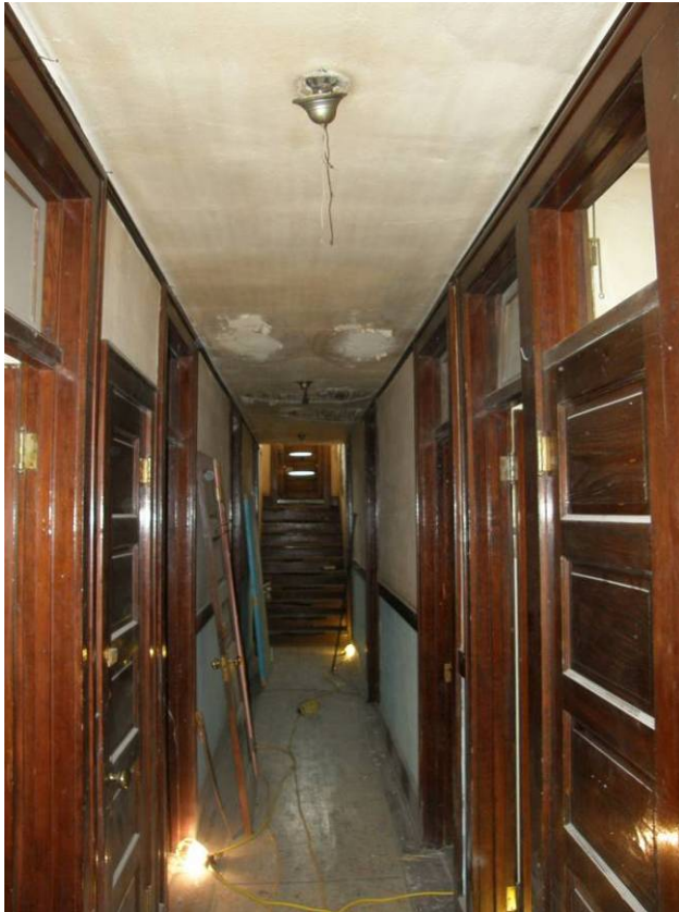
Main corridor looking south from skylight to lower roof access stair
