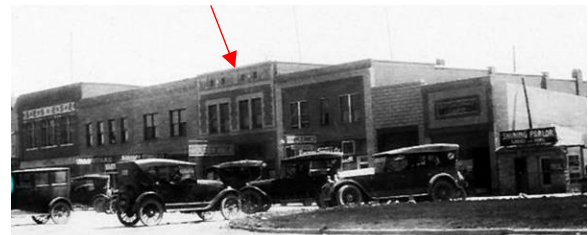
Circa 1916 Streetscape: The Golden Rule Store (center building)
