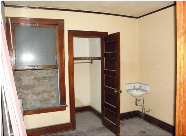
Room #10 looking east to closet & light well
