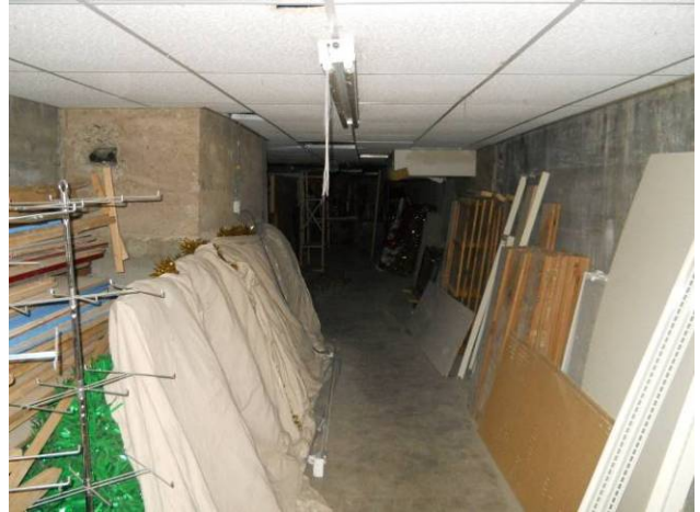
Main hall looking north
