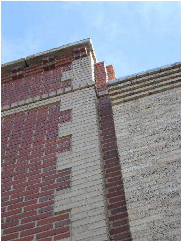
Corner detail of brickwork at second story, North façade, West edge
