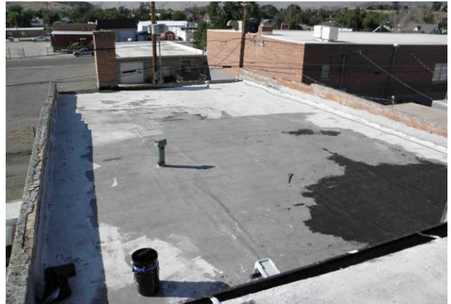
Lower roof looking southwest
