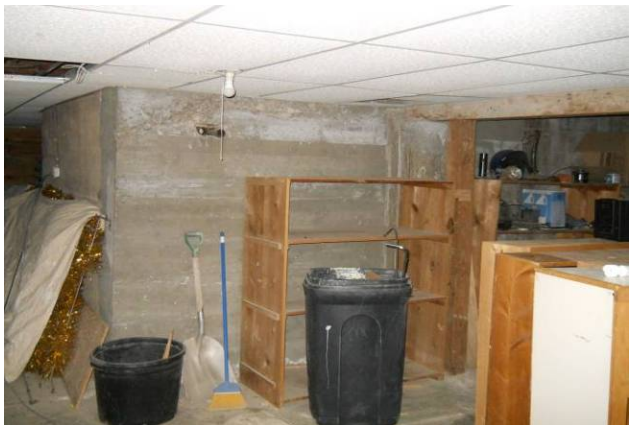
View of previous building foundation walls looking south
