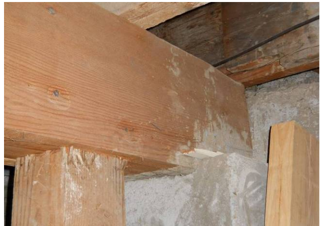
Structural floor beam connection into foundation wall
