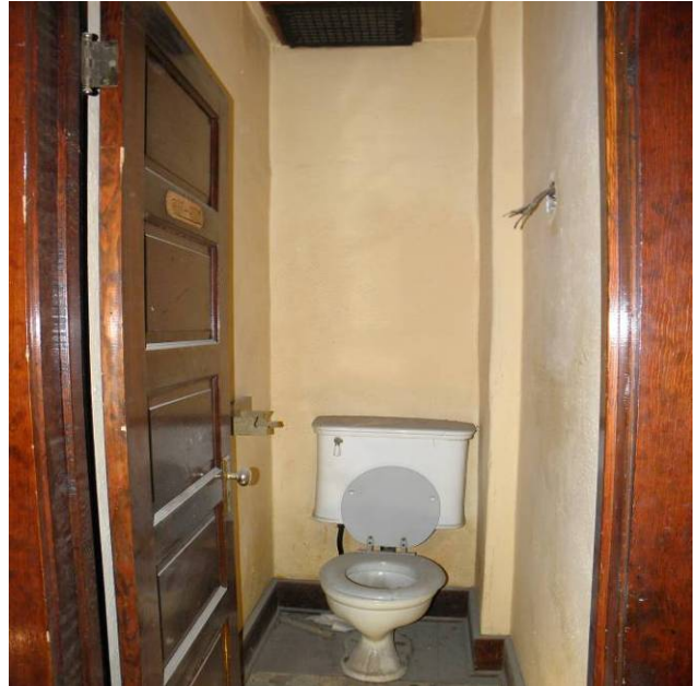
Single restroom adjacent to utility sink, looking west
