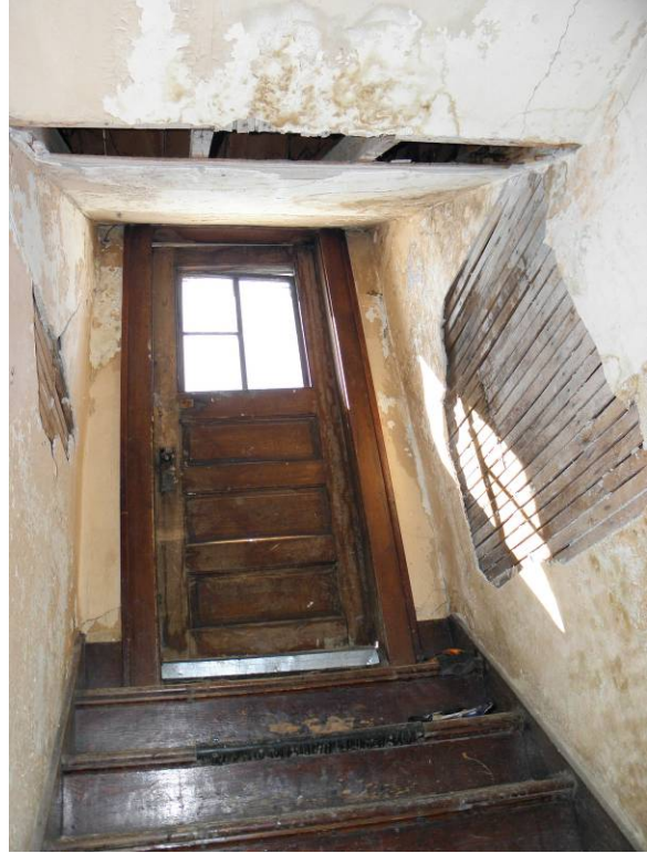
South door from second floor to roof
