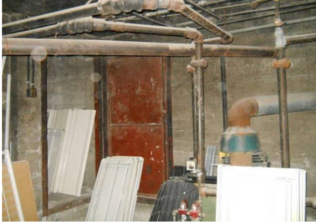
Boiler room – looking back at entry door/north
