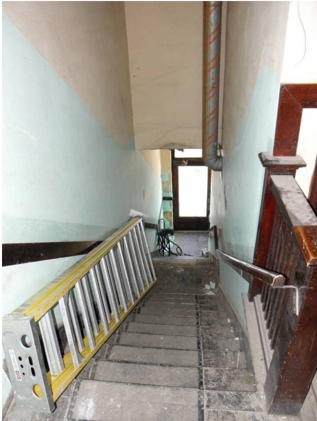
Stair looking north to 1 st floor entrance
