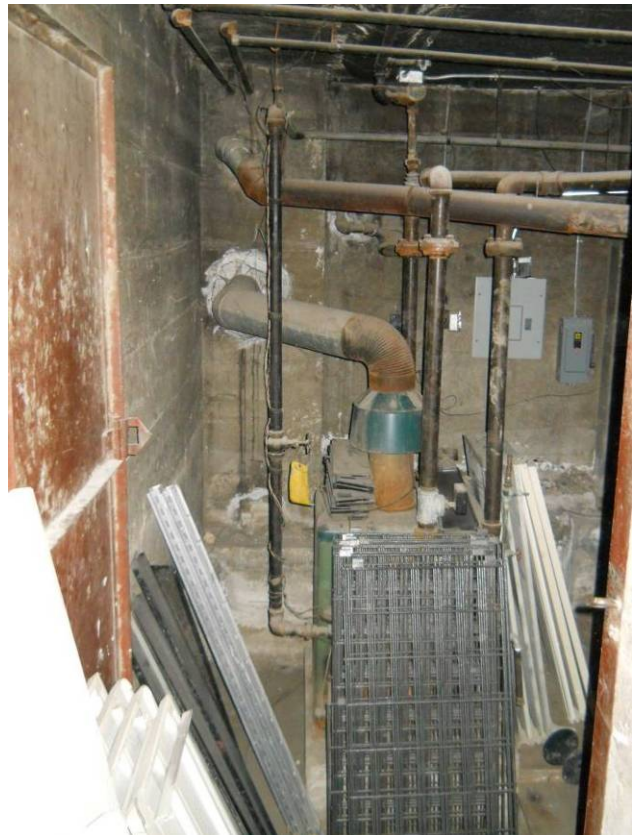
Boiler room looking south
