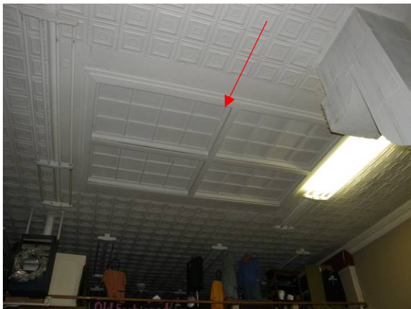
View of south skylight location, covered up over roofed over
