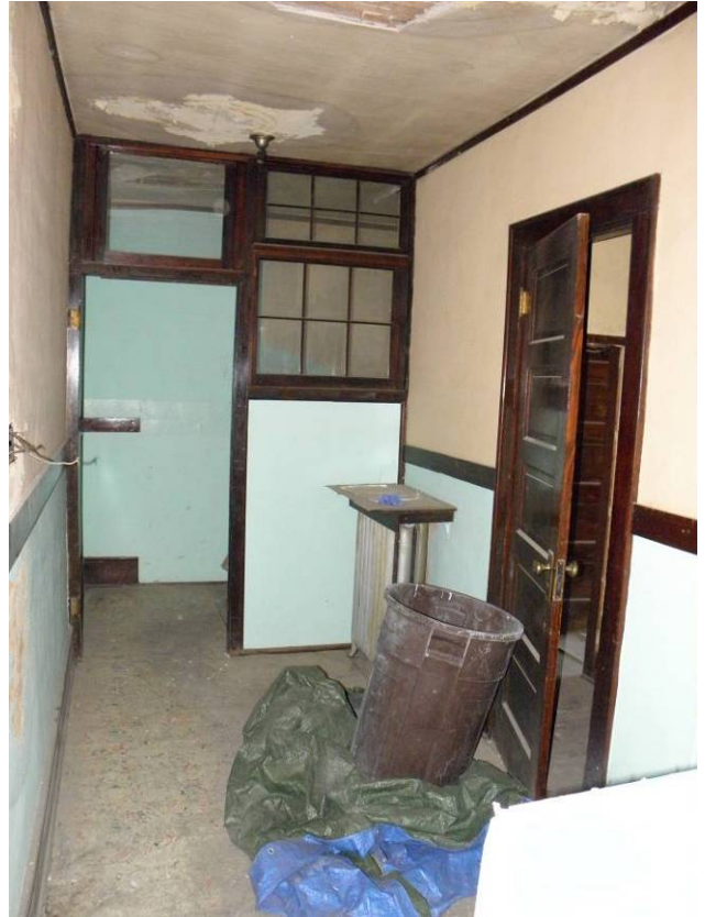
Entry corridor beyond stair landing, looking west
