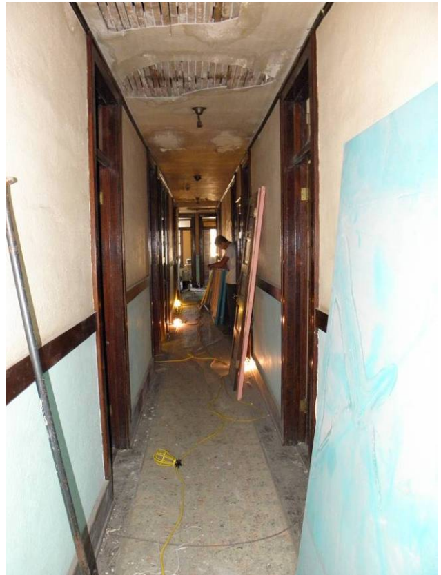
View of corridor looking north from south stair
