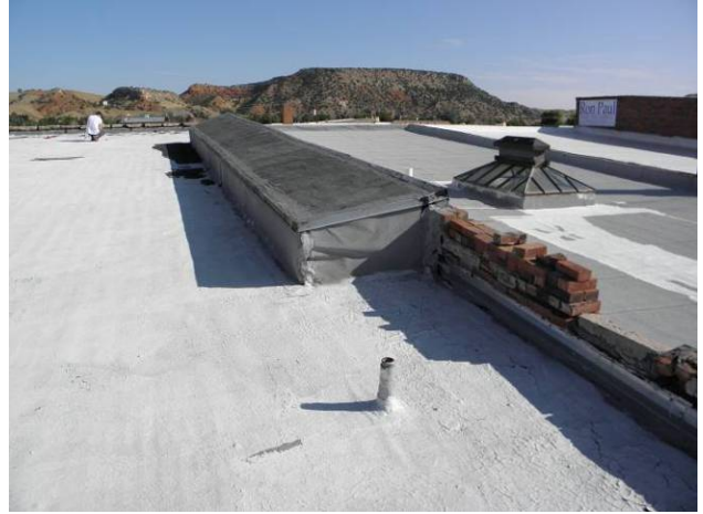
View of East lightwell looking Northeast
