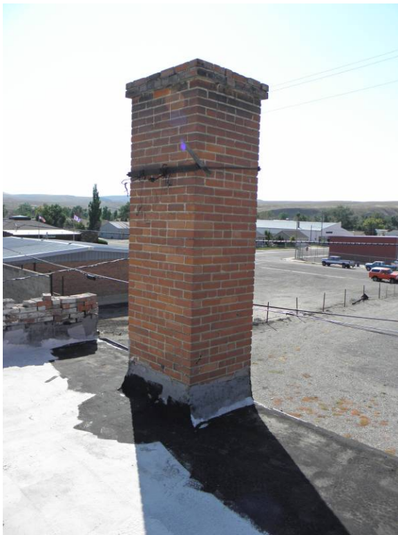
View of south chimney on lower roof
