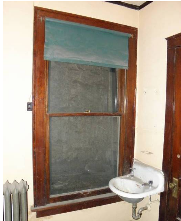
Typical east/west window
