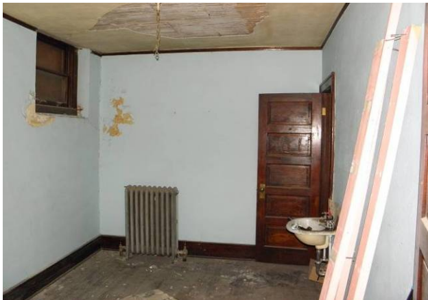
Room #11 looking west
