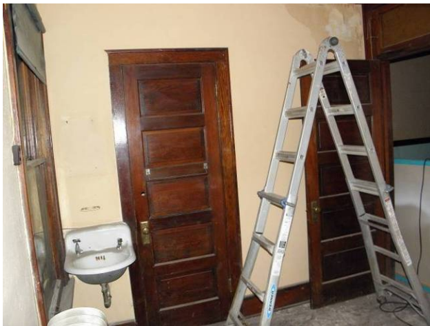
Room #3 looking south to closet
