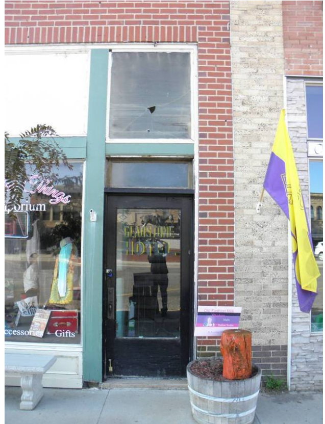
Second Floor Hotel entry door
