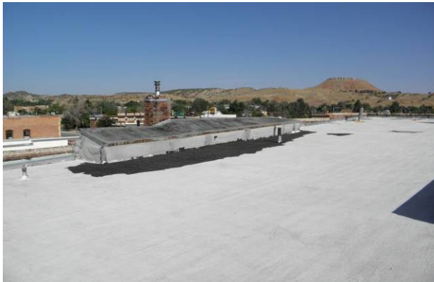
View of West lightwell looking Northwest
