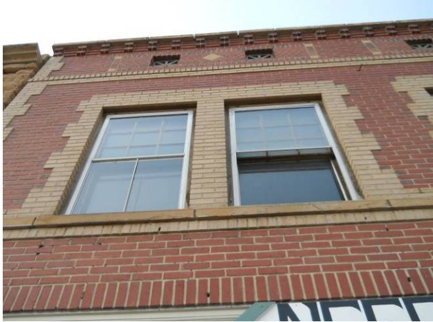
North façade upper windows
