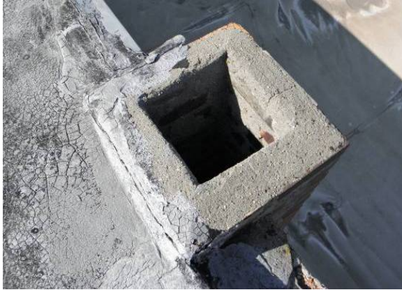
View of northwest chimney on upper roof
