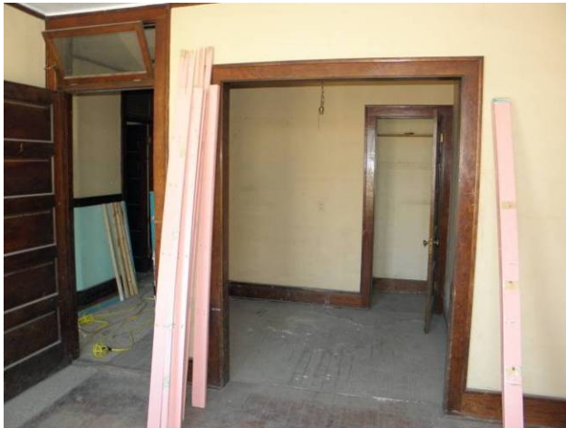
Room #1 looking southeast toward main corridor
