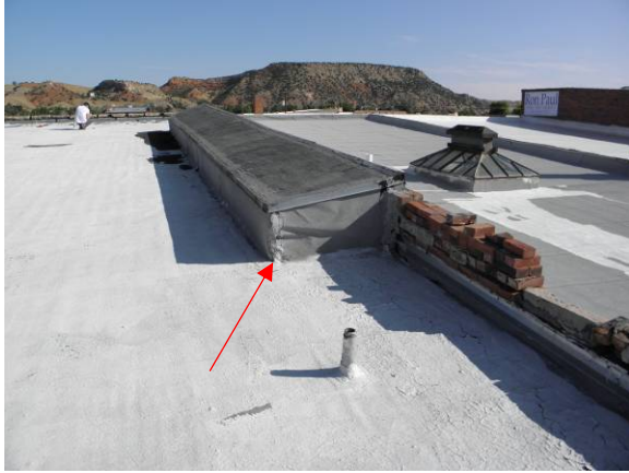
View of covered light well on east side looking north
