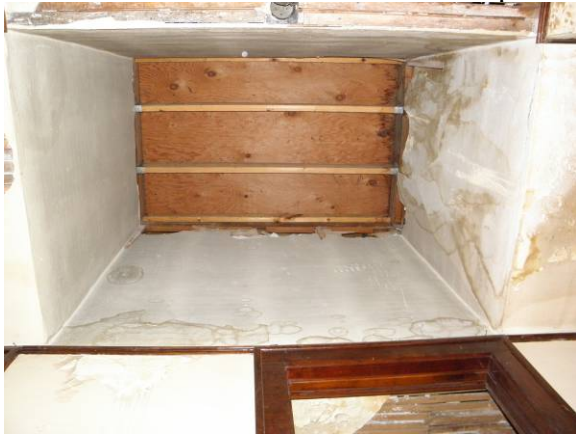
View of north skylight location, currently covered up and roofed over
