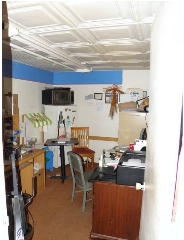
Administrative office under mezzanine & adjacent to stair, looking south
