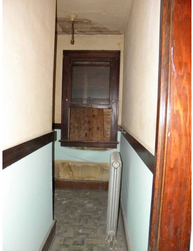
Bathroom adjacent to Room #5, looking west, window into light well beyond
