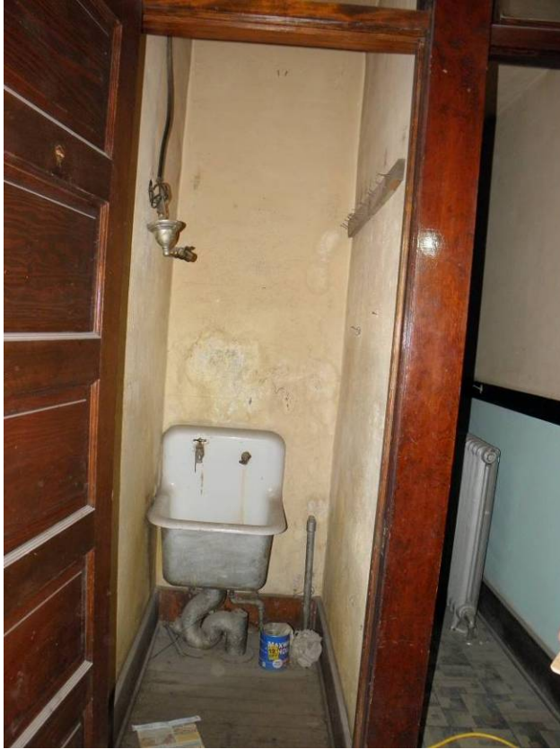
Utility sink closet adjacent to restroom, looking west
