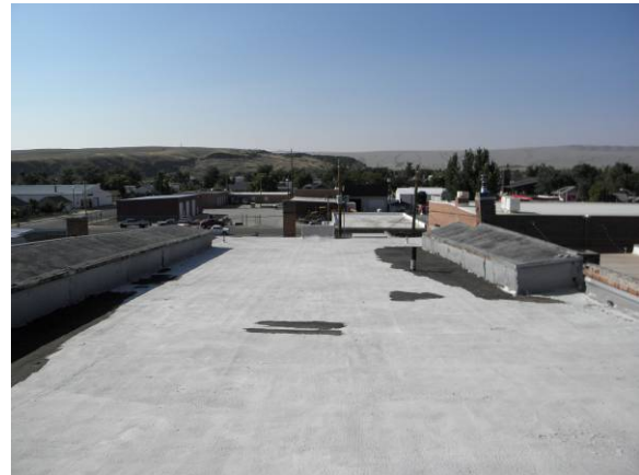
View of upper existing roof looking south
