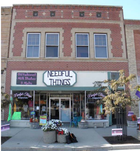
2015: View of current north façade
