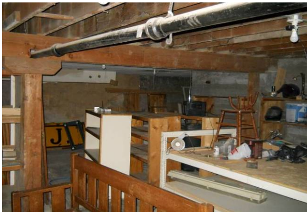
Central storage looking southeast
