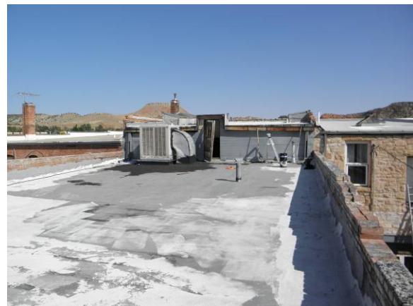
View of lower existing roof looking north
