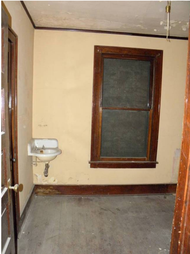
Room #8 looking east to light well
