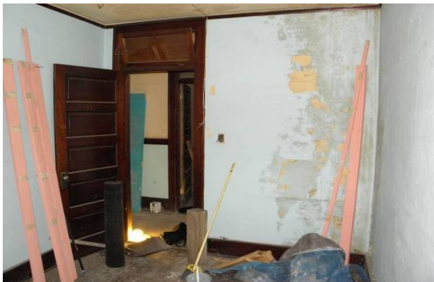
Room #11 looking east to main corridor
