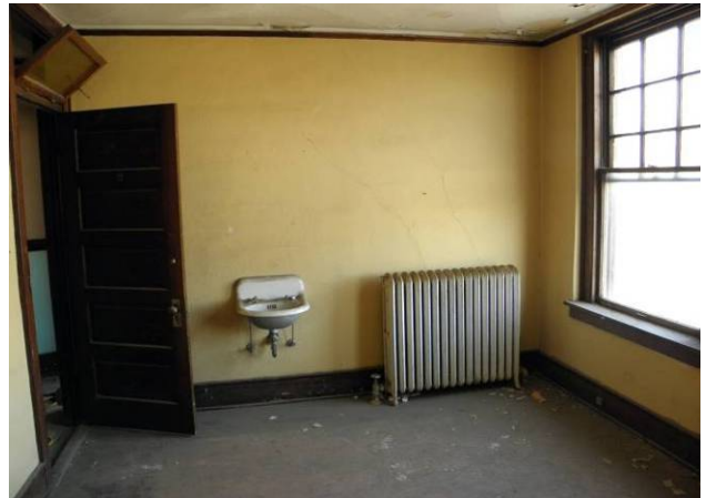
Room #2 looking west, interior corridor on left, Broadway Street on right outside window
