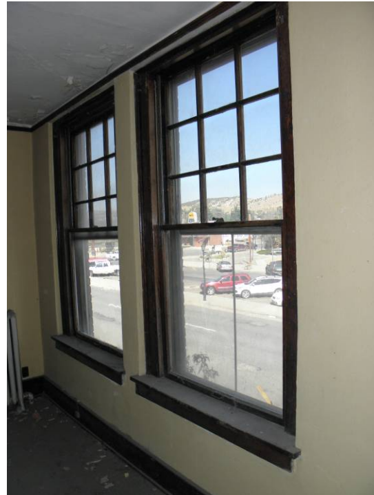
View of north windows
