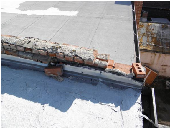
View of an upper east brick parapet
