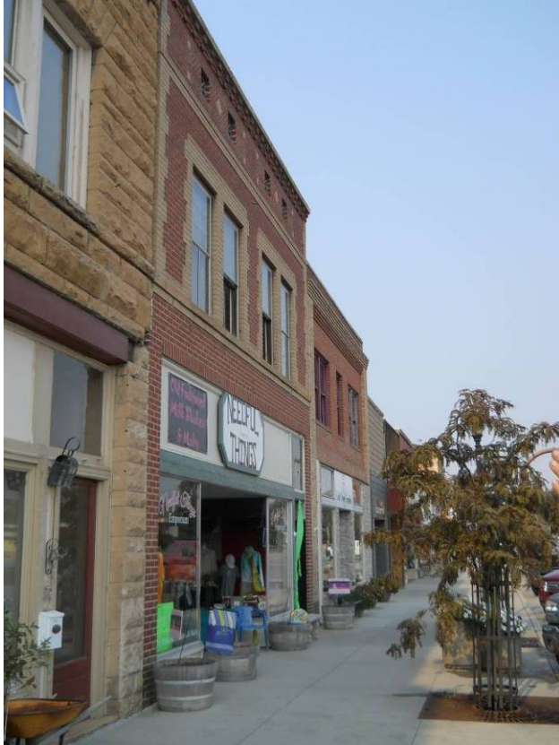
North façade looking West
