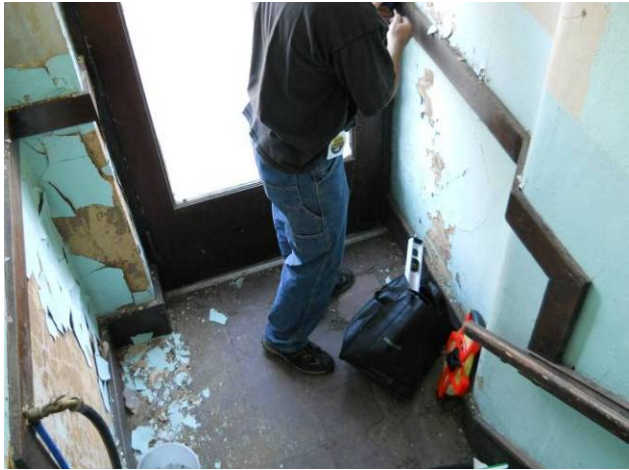
Street entrance to second floor stair, looking north
