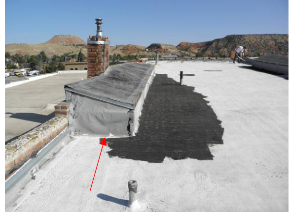
View of covered light well on west side looking north
