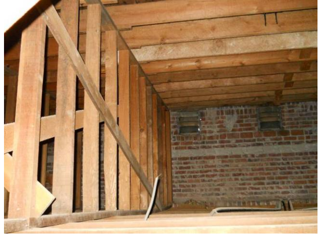
Attic space above rooms at north end looking north
