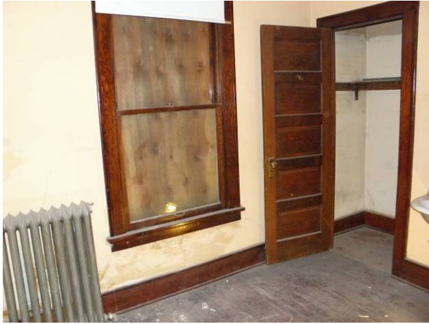
View of west wall & closet, Room #7
