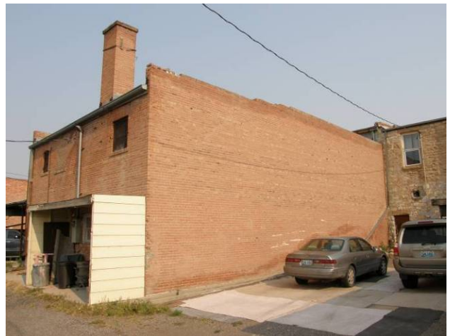
Southeast corner looking Northwest
