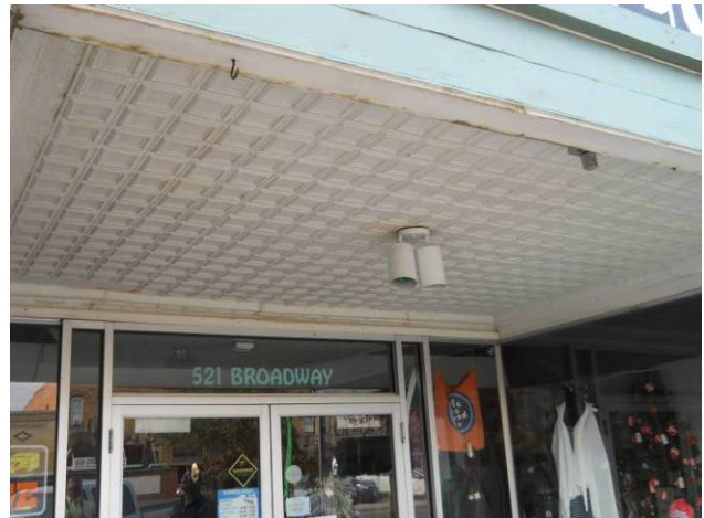
Existing entrance and tin ceiling
