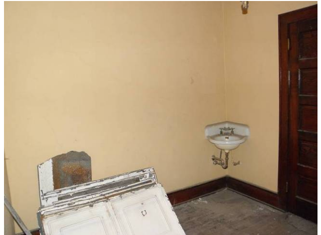
Room #9 looking southwest
