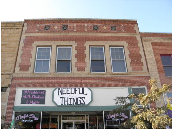
View of north historic facade fronting Broadway
