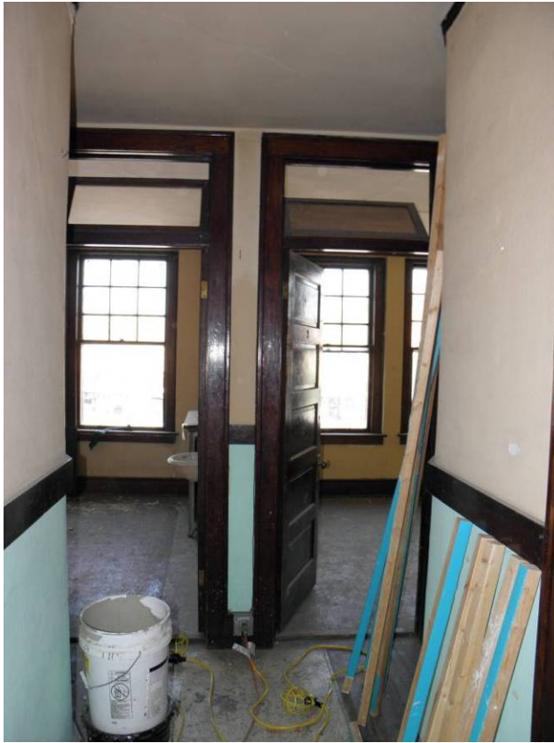
Main corridor looking north from entry area
