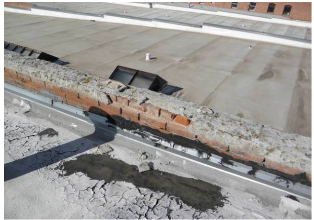
View of West parapet wall, looking West
