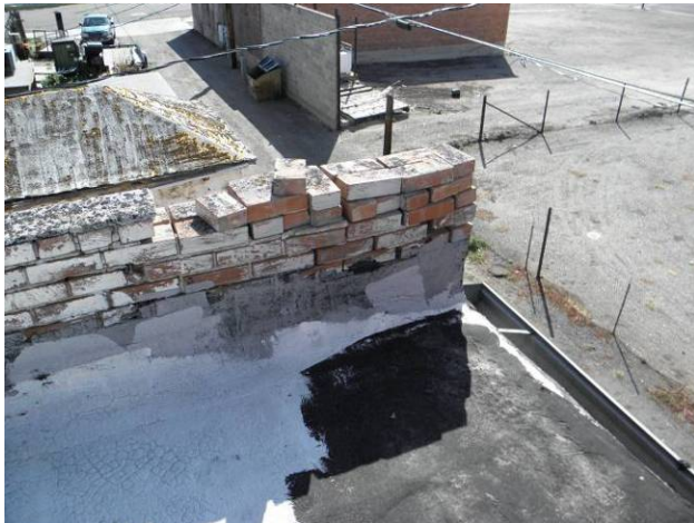
View of southeast parapet
