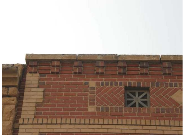
Decorative attic venting and brick detailing, North façade
