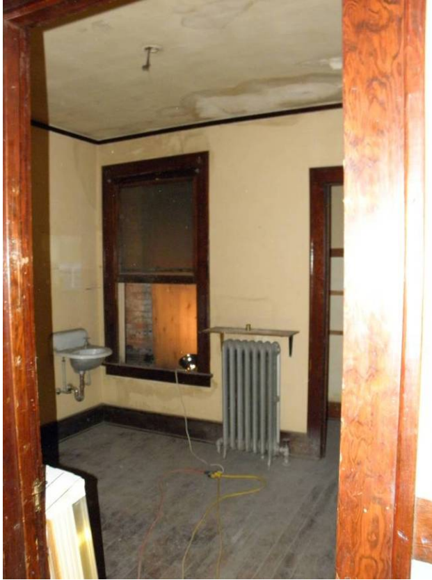
Room #5 looking west to light well
