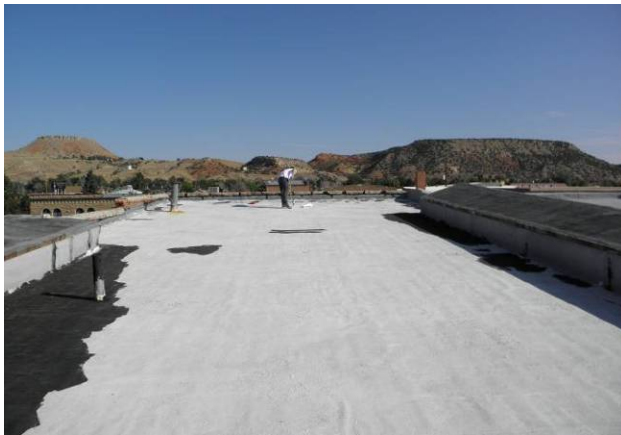
Upper roof looking North
