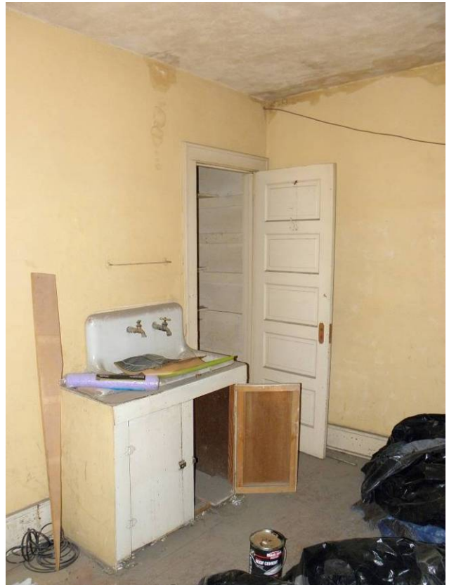
Room #12 looking northeast to closet
