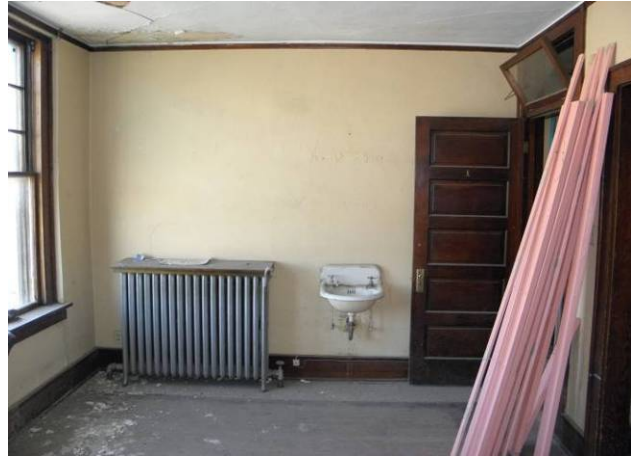
Room #1 looking east
